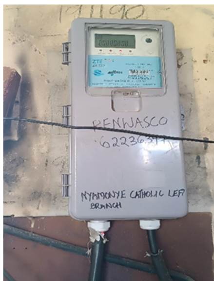
Figure 4. 3-phase meter at the pump house
