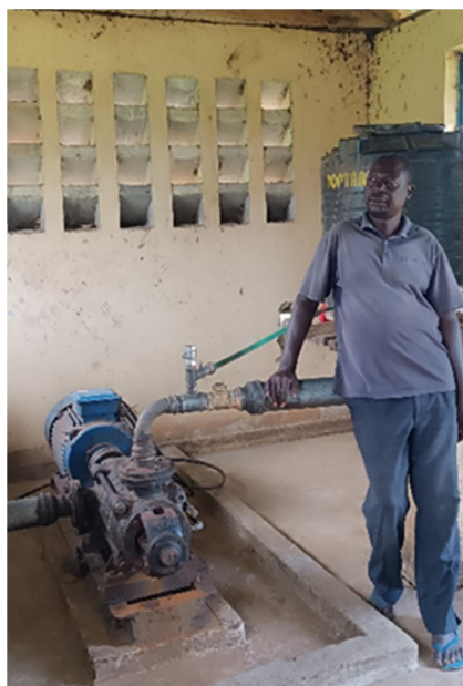
Figure 3. Pump house energized by grid electricity
