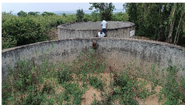
Figure 2. The sand filtration tank
